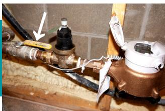
Older meters may have turning handles. Most have valves on either side of the meter. Turn them both off before leaving.
