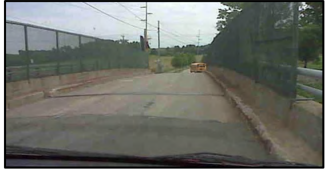
Powell Road Turnpike Bridge
