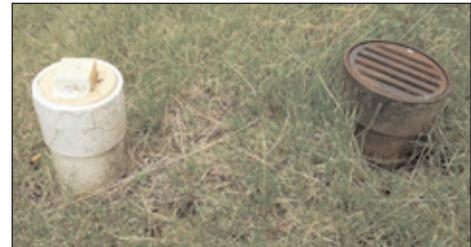
***Down the drain.*** Every home connected to the Township's sanitary sewer system has a fresh air vent and a cleanout port, like these. If they're blocked, broken, missing, or too low to the ground, they can act like storm drains, leading to serious capacity problems for the sewage treatment plant.
