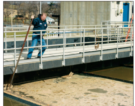
Scum of the earth. Fats and grease sent down the drain create foul odors adding to the cost and difficulty of sewage plant operation. Here, veteran wastewater plant worker Walt Koach opens a valve to skim off the surface grease accumulated over a four hour period at the Brush Creek facility.
