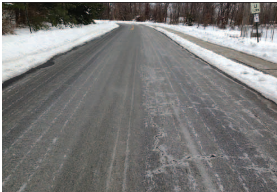
Telltale stripes. Salt brine is sprayed and then dried onto the road surface before a snow storm to prevent icing.
