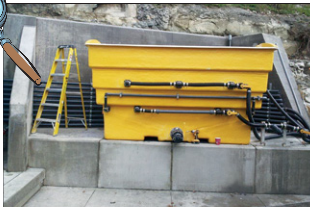
Secret brew. This computer-controlled mixing vat is capable of producing up to 3,000 gallons an hour of precisely calibrated brine for application by Township salt trucks.
