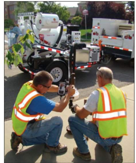
Public Works field operators Rob Caughey and Curt Rape use the department's new valve maintenance trailer to exercise water valves recessed into a residential driveway.
